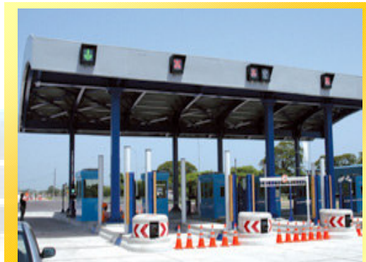
Highway 2000 Toll Plaza
