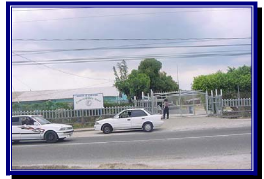
Crescent Primary School – one focus of the 2004 Labour Day Project
